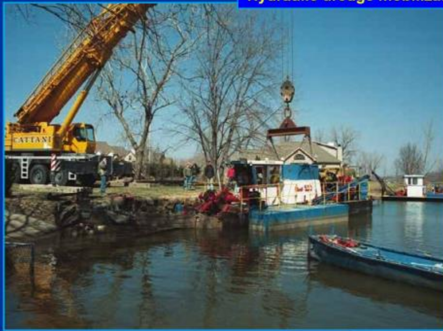
Hydraulic dredge mobilization and pipeline assembly.
