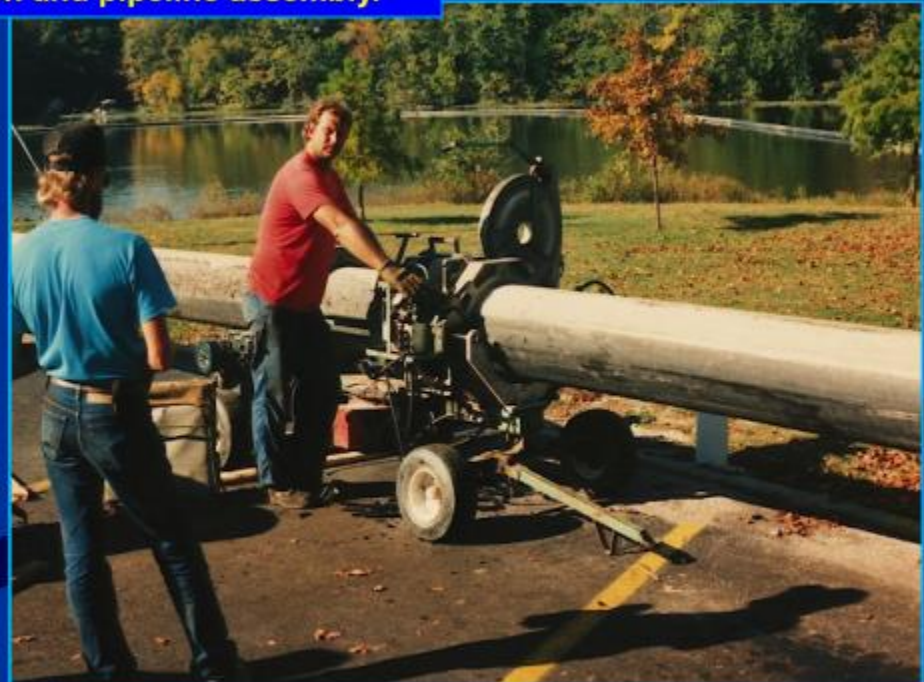
Hydraulic dredge mobilization and pipeline assembly.
