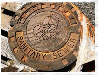
Waste water flows through the main sanitary sewer lines by gravity and force from lift stations to a wastewater treatment plant where the wastewater gets treated.
